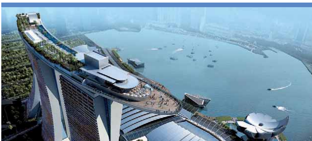
Marina Sands Bay, Singapore (44.000 supporti SE3 - SE7) Marina Sands Bay, Singapur (44.000 pedestals SE3 - SE7) Marina Sands Bay, Singapor (44.000 soportes SE3 - SE7)
